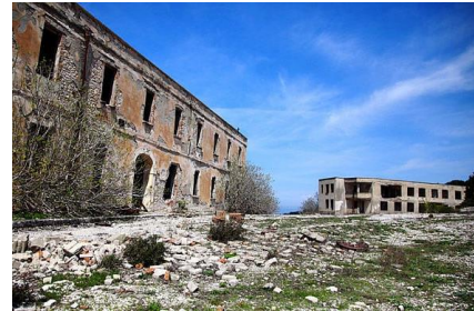
Abandoned military barracks Sazan
